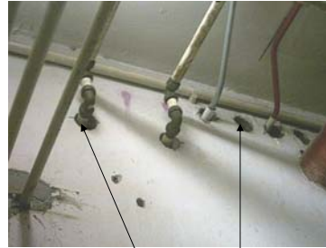
Holes on wall without proper sealing up
